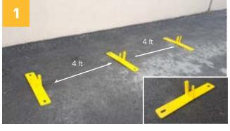
All Modu-Loc fence bases consist of one square and one round peg. Lay out fence bases 4ft apart with all of the round pegs facing the direction you will build your fence.
