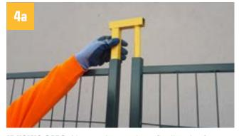
IF USING CAPS: Now you're ready to finalize the fence set-up by installing the caps. All the caps also consist of one square and one round peq. These need to be installed in the same fashion that the bases were laid out: round peas line up with round peas and square with square. Insert the cap into the top of the panel, and slide the cap in completely.
