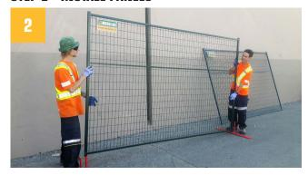
With a partner, begin assembling the fence panels onto the bases. Insert the square peg into the panel first, then drag the panel back to the previously installed base and place it on the round peg.
