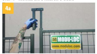
IF USING CAPS: Now you're ready to finalize the fence set-up by installing the caps. All the caps also consist of one square and one round peg. These need to be installed in the same fashion that the bases were laid out: round peas line up with round peas and square with square. Insert the cap into the top of the panel, and slide the cap in completely.
