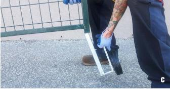
Gates can be installed anywhere in the fence line. Gates swing on the round peg. When installing a gate, place one spacer over the round peg (a) before placing the panel onto the base (b). This will elevate the panel and allow the gate to swing freely. Install the wheel at the opposite end of the panel (c). With the spacer and wheel installed, the gate should be level and swing freely.
